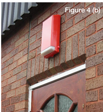
Figure 4: External sounders should be installed at high level, eg 4m above ground, as shown in (a), not (b)
